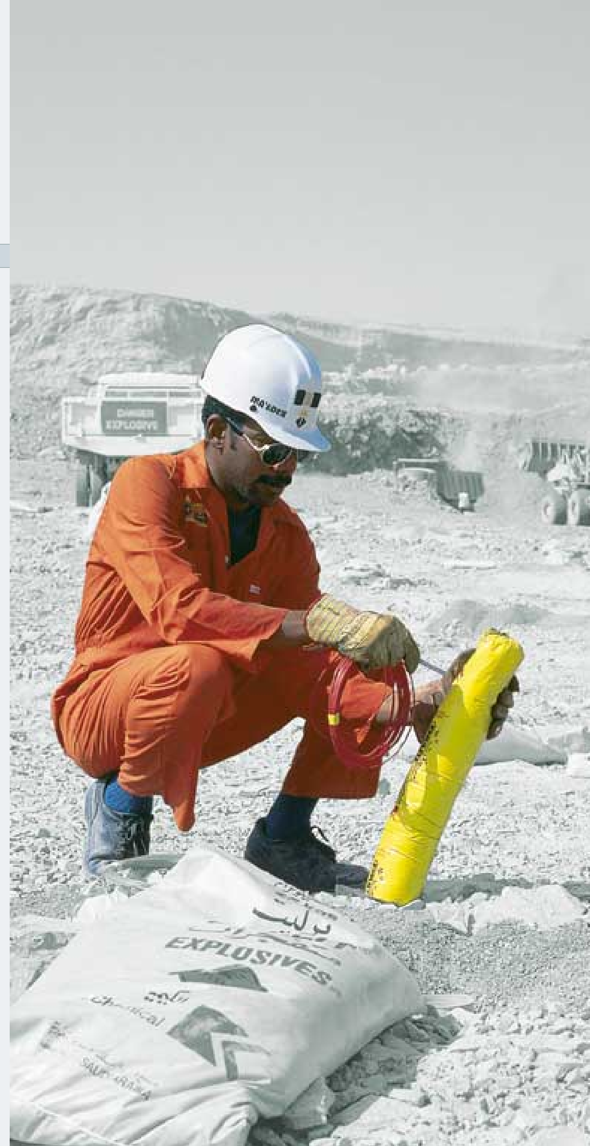
Setting charges for pit development
