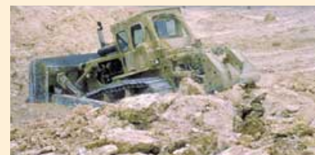
Clearing overburden at Al Jalamid
