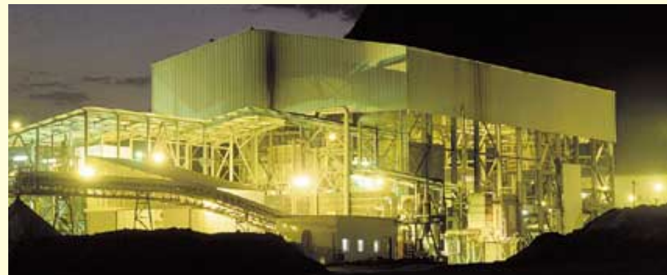
Processing plant at the mine
