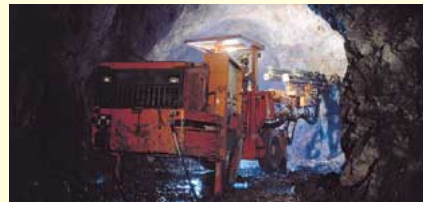
Jumbo drilling production holes underground
